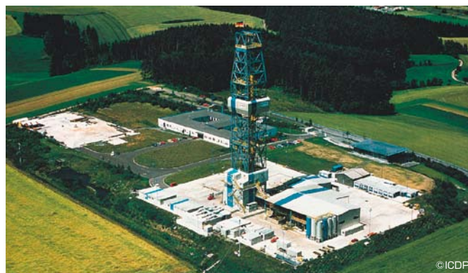
The German Continental Deep Drilling Program (KTB), which was instrumental in establishing the ICDP. The main bore (approx. 9 km) and pilot bore (approx. 4 km) are currently still used for ICDP experiments.
